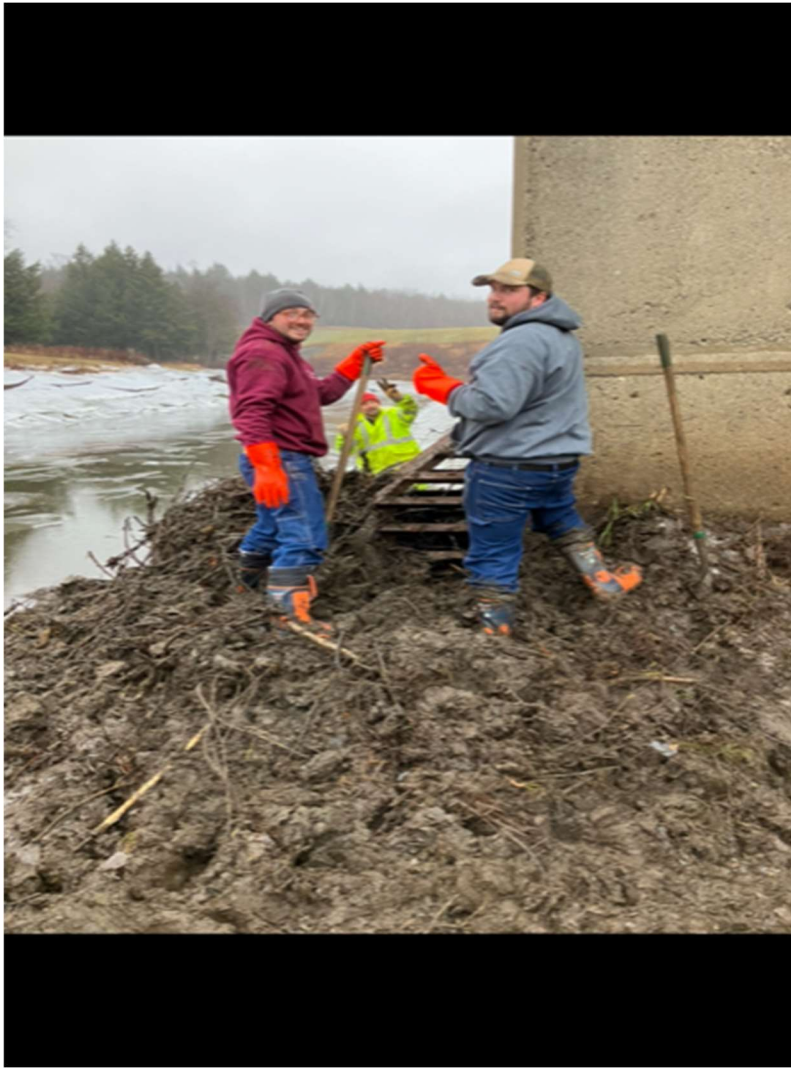
Water Dept Crew – Beaver Dam Dig-out Photo by Joe Gaudiana, Chief Operator
